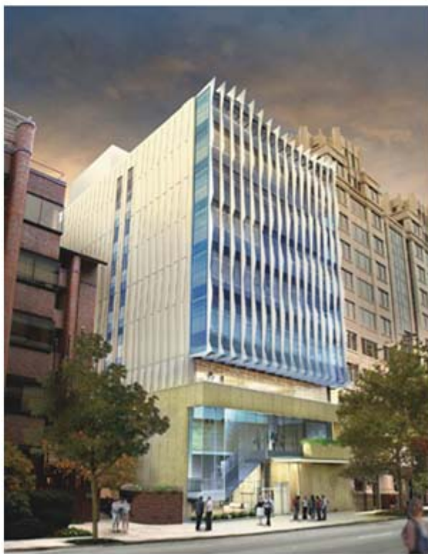
Courtesy Hickok Cole Architects
