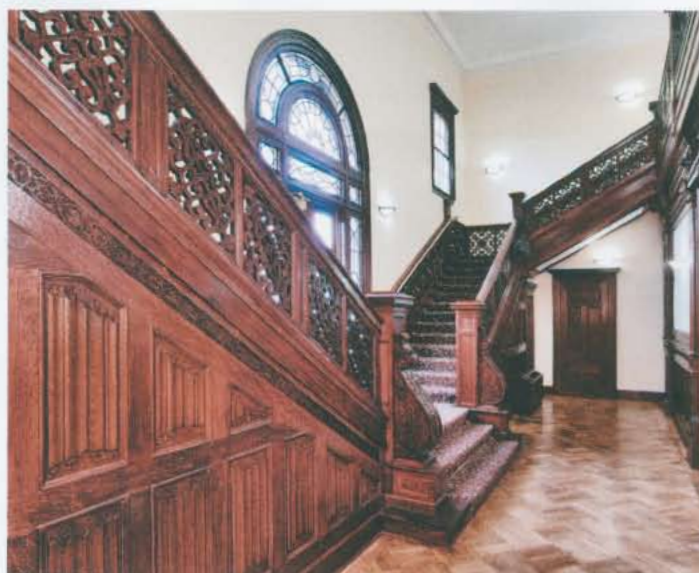
Top: The lobby at CASA de Maryland's new center is made of oak linenfold panels. The alcove near the fireplace was burned out before the restoration. Bottom: The original hand-carved oak staircase, with new brass rails, leads to the second-floor offices.
