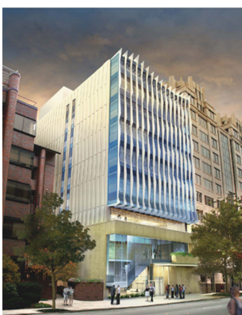
Rendering of the New York University Constance Milstein and Family Academic Center designed by Hickok Cole Architects
