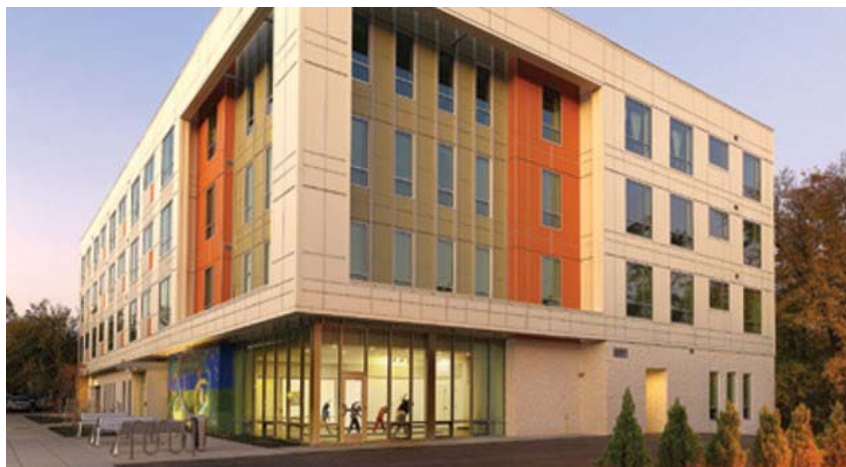
Brookland Artspace Lofts.
