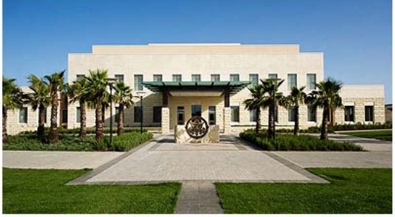
The new U.S. Embassy compound in Valletta, Malta, designed by KCCT , has been completed. Photo: Alan Carville Extra Large Image
