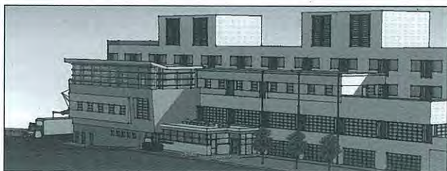
National Rehabilitation Hospital's Second Floor Addition
